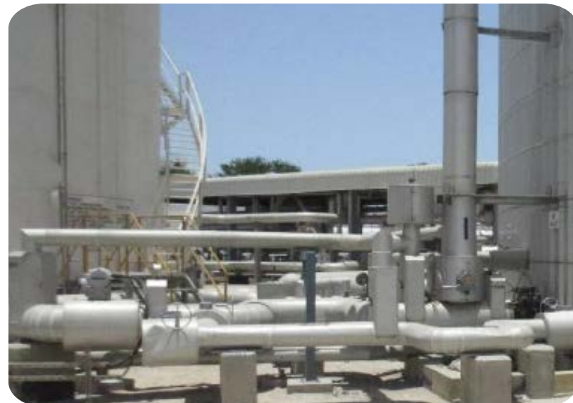
TANK FARM CLADDING AND INSULATION
