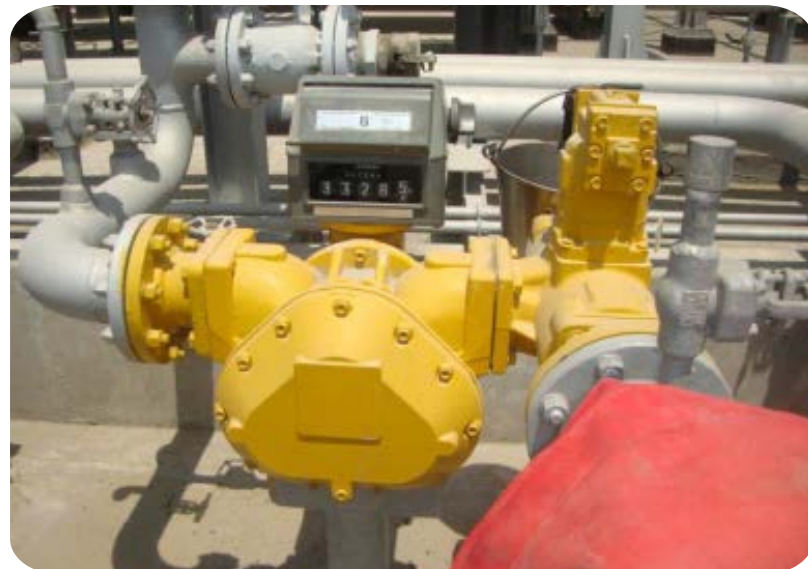
FLOW METER INSTALLATION
