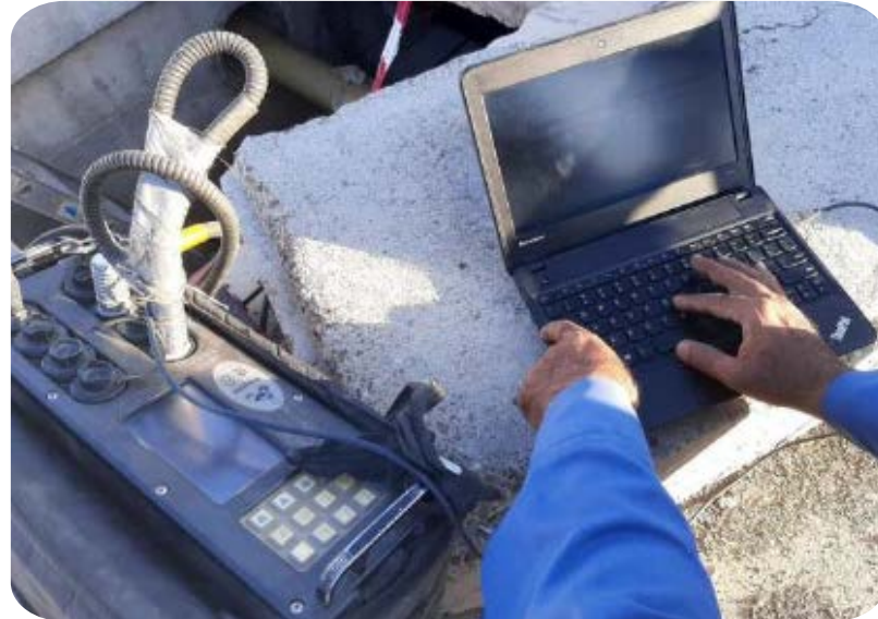
INSPECTION OF EQUIPMENT MEP
