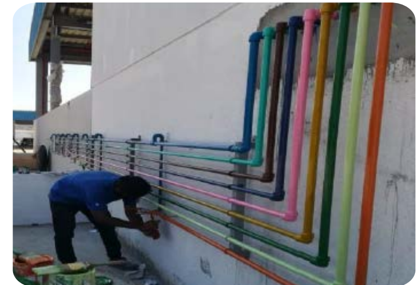
INSTALLTION OF UTILITY LINES
