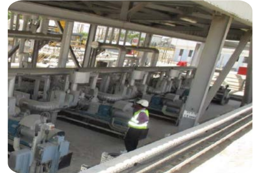
PUMP HOUSE INSPECTION
