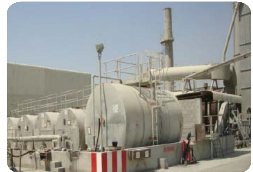
BITUMEN FACILITIES INSPECTION
