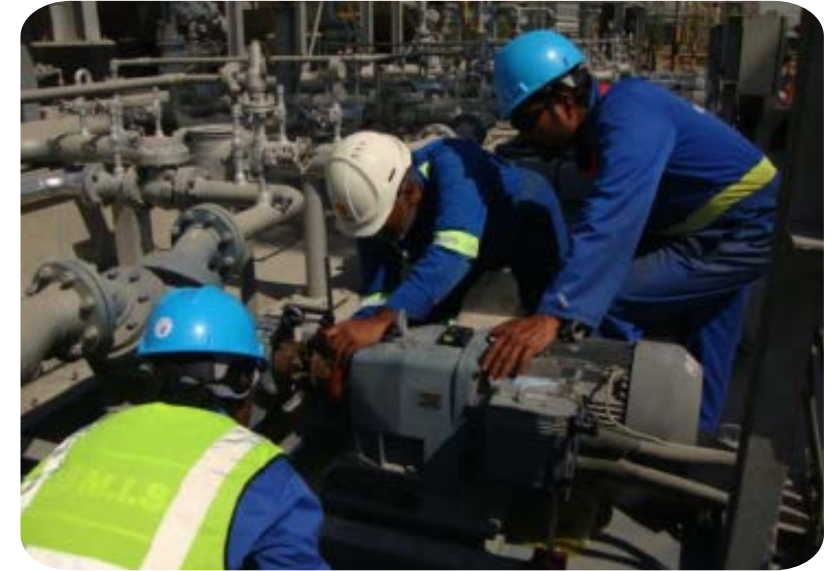
PUMP INSPECTION & MAINTENANCE
