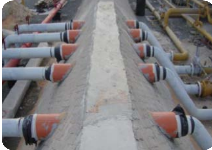
SITE EXECUTION - PIPING
