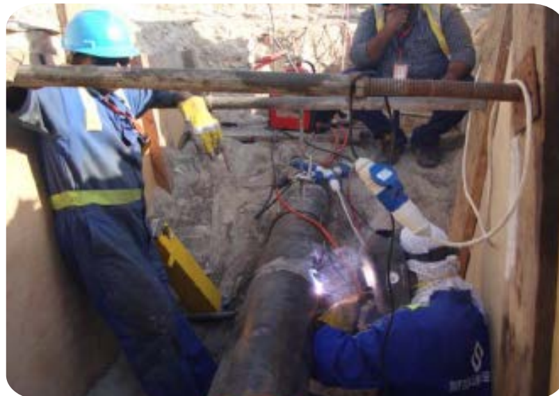
UNDERGROUND PIPING WORKS
