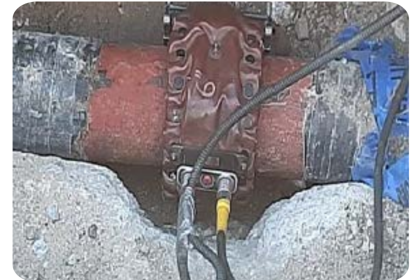
LRUT INSPECTION OF UNDERGROUND PIPING
